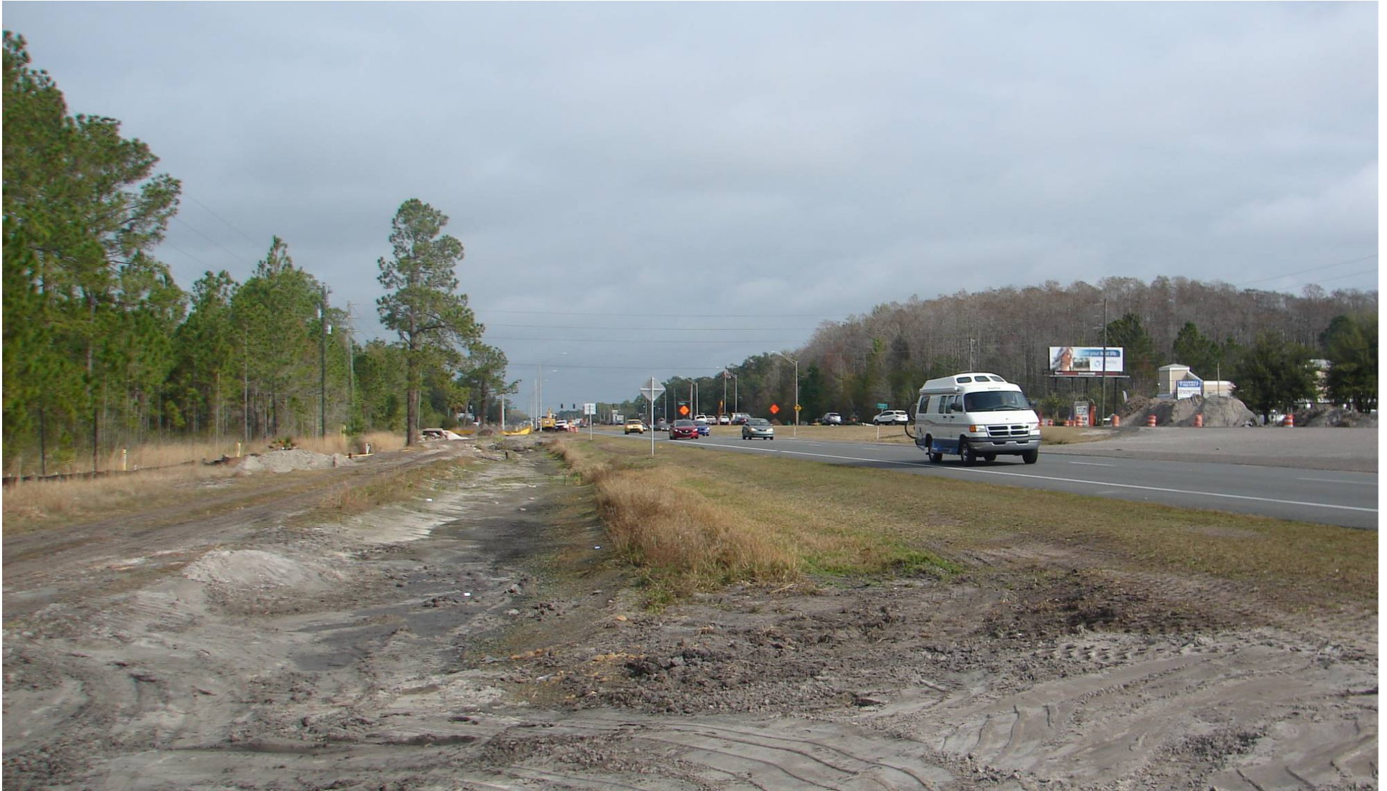
Attachment: Coordinator's PowerPoint (20535 : CU-22-04 Michael Wilburn for Acme Storage)
