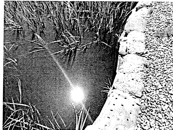
Photo 6. A photo of a culvert under the driveway crossing through a tidal stream on-site.
