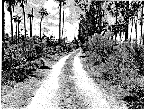
Photo 2. A photo of the winding limestone base drive access present on-site.
