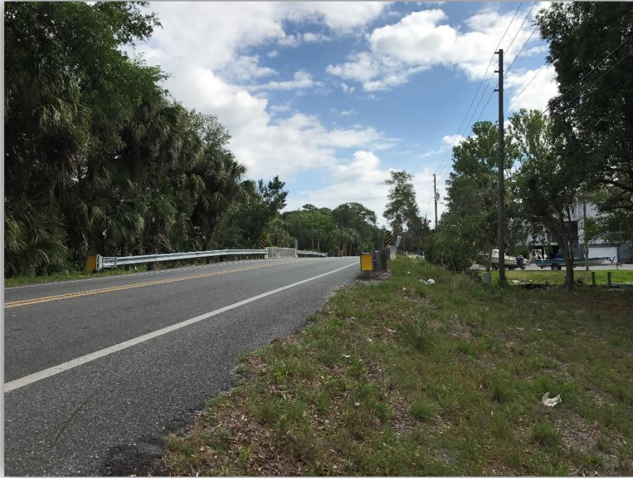
Canal Crossing under Fort Island Trail
