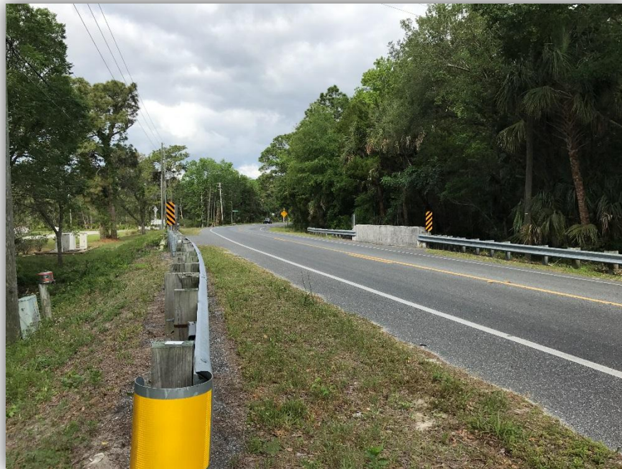
Canal Crossing under Fort Island Trail
