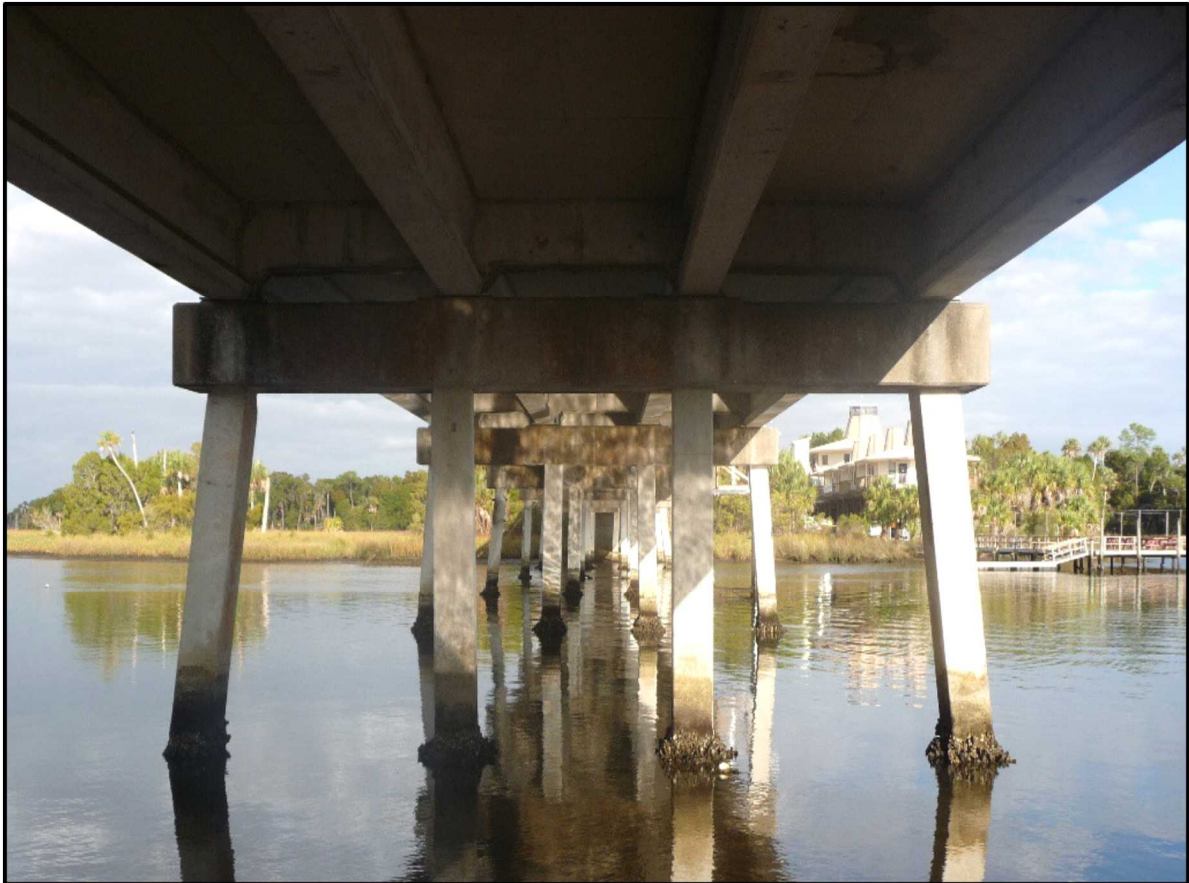
Photograph 2 - Salt River Bridge structure
