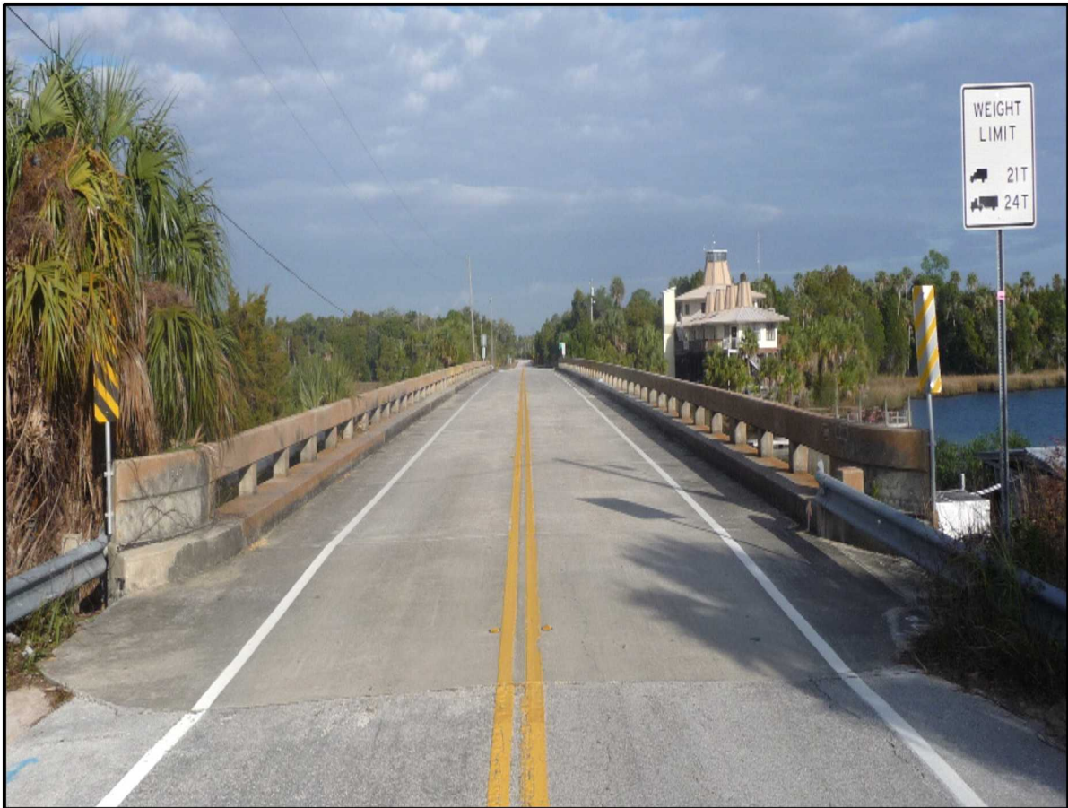
Photograph 1 - Salt River Bridge, looking west from east
