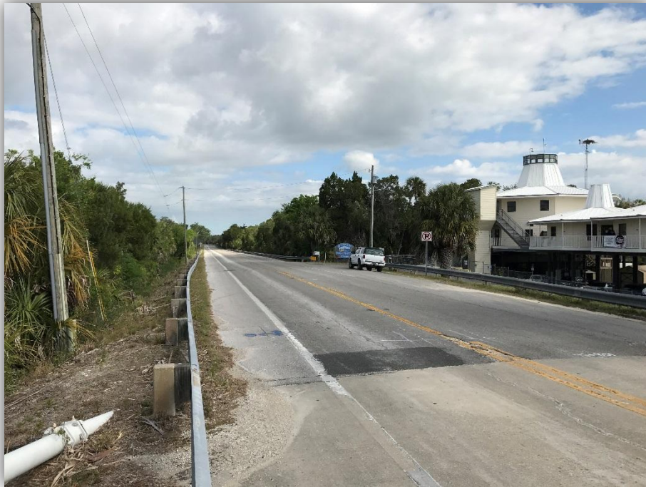
Looking west along the Salt River Bridge, towards the Academy of Environmental Science
