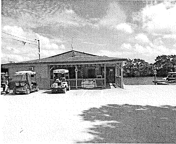
Front view of Marina/Grill Room
